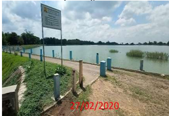
Figure 3. Condition of Inundation Area
