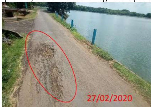
Figure 1. Condition of the Dam Top
