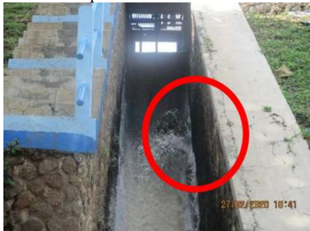
Figure 5. Condition of the Spillway Building
