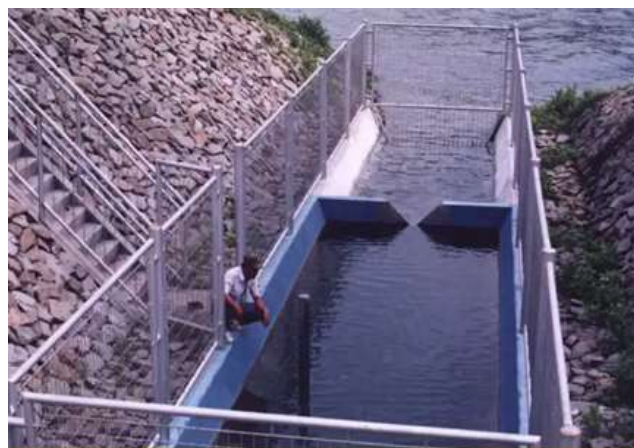
Figure 7. V-notch Shape of the Dam
