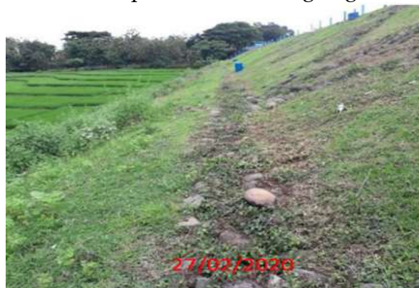
Figure 2. Condition of Dam Slopes
