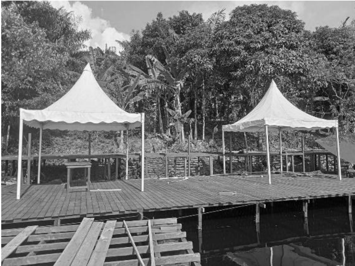
Figure 2. Langit Timur Pier Construction Process
