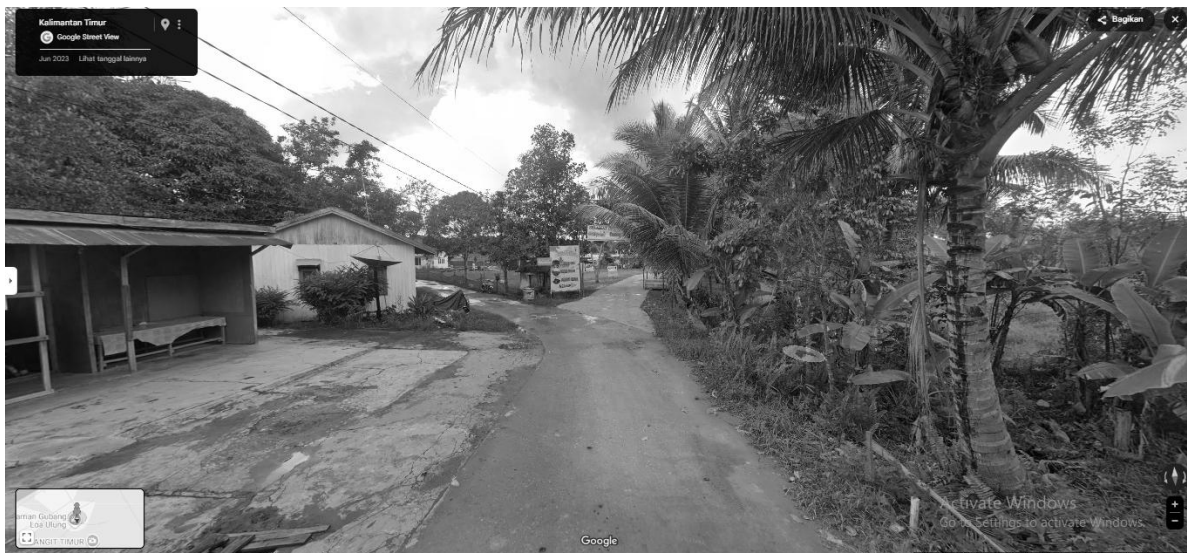
Figure 3. Road Conditions to the Tourist Attraction Source: Google Street View, 2025
