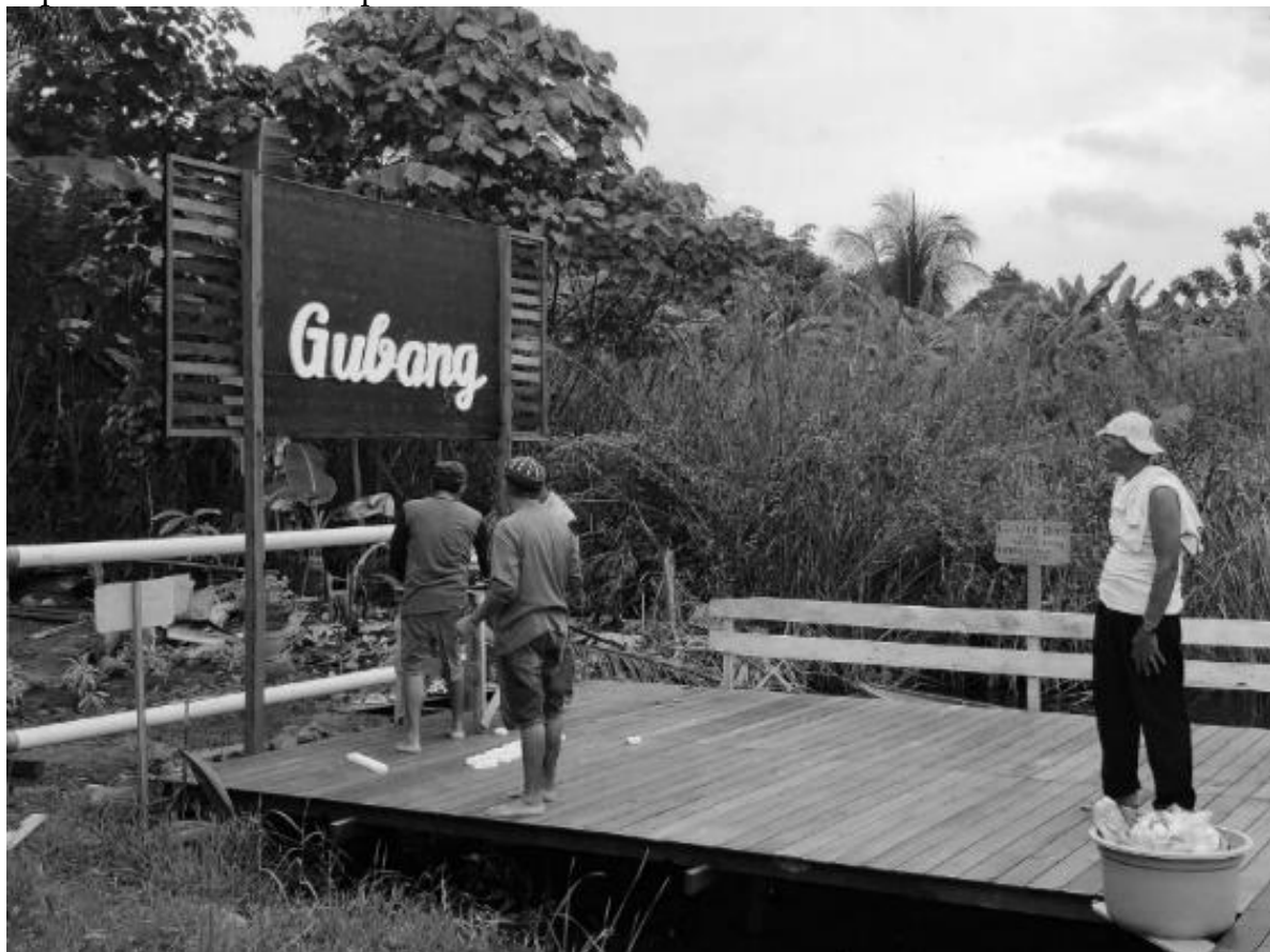
Figure 1. Taman Gubang Pier Construction Process
