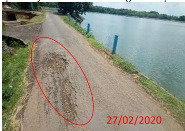
Figure 1. Condition of the Dam Top
