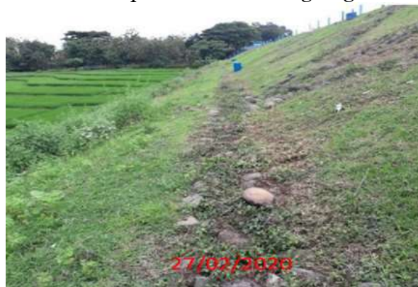
Figure 2. Condition of Dam Slopes
