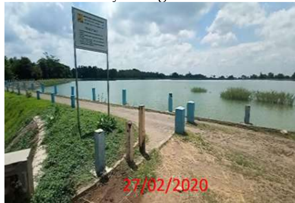
Figure 3. Condition of Inundation Area
