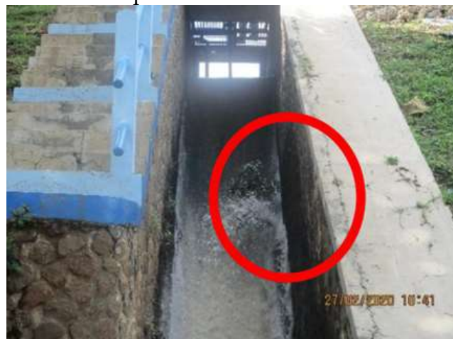
Figure 5. Condition of the Spillway Building
