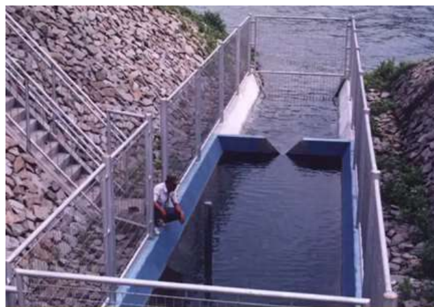
Figure 7. V-notch Shape of the Dam
